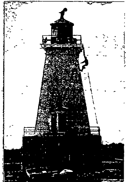
A painter sits suspended on a bosun's chair at Sandy Point, October 2002
