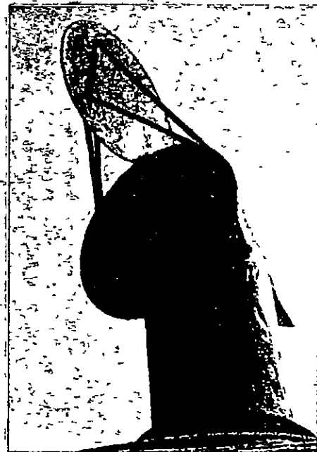
A weathered ventilator sits atop the Sandy Point lantern
